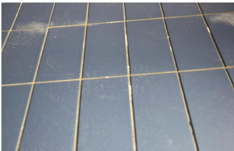
Experience shows that almost all pools where the tiles have loosened, have had a water quality with a LSI index indicating *very aggressive* or *moderately aggressive* water. We have thought that if the joint grout is intact they will protect the adhesive against aggressive water and that the risk of chemical attack of the adhesive is small.
